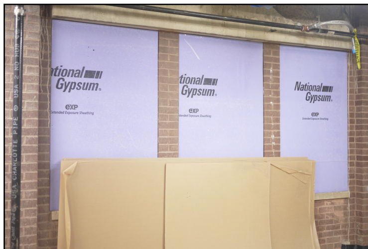
figure4. demolition place between SPT and ETB
