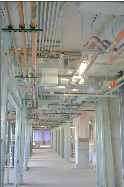
figure1. BIM coordinated MEP system
