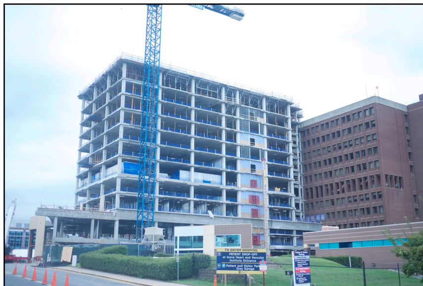
figure3. SPT tying to ETB
